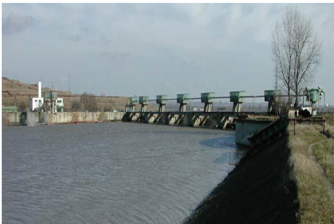
Figure 2. The Işalniţa water intake dam (original).
